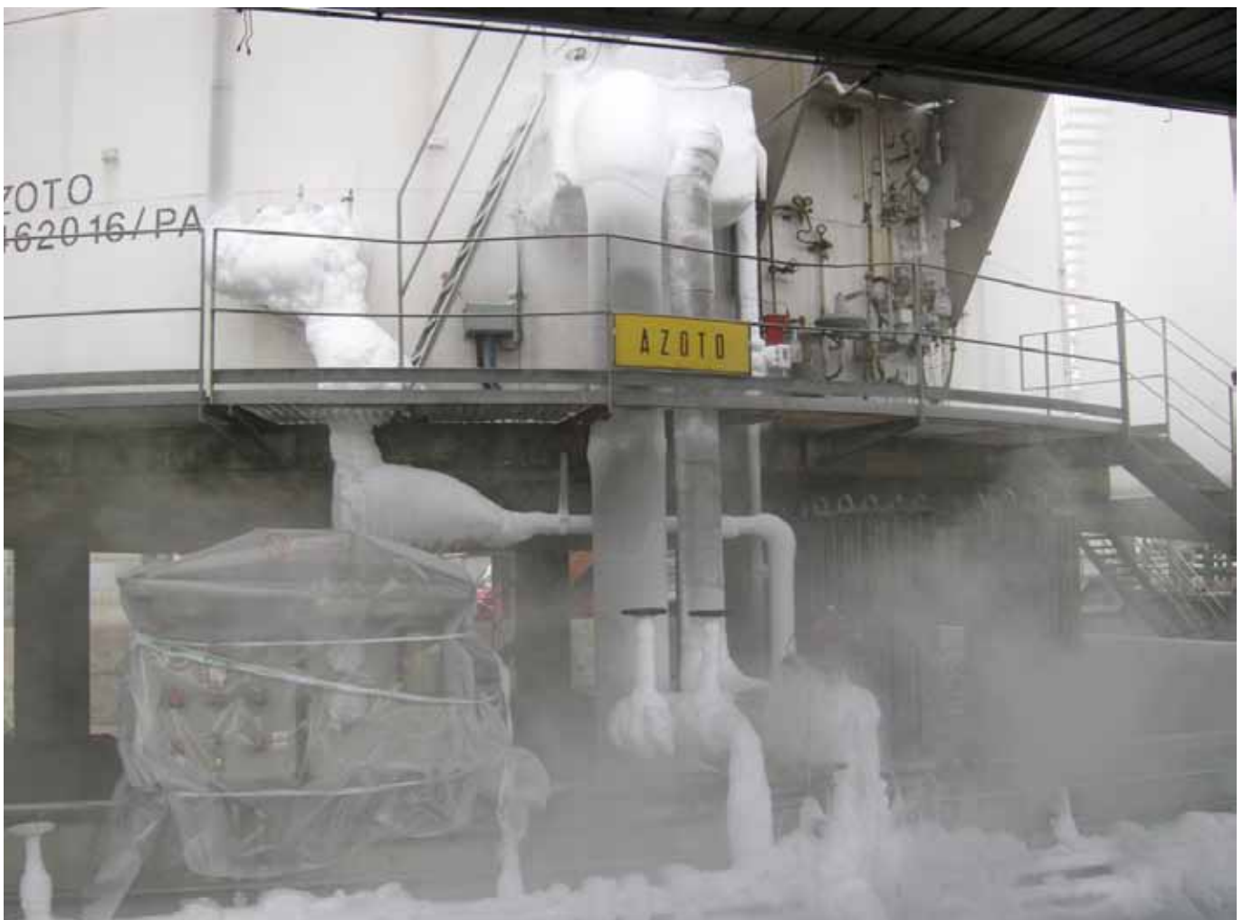
Figure C-10 Control panel needed to be protected with plastic sheeting from the dripping condensation water. Extensive ice building on pipes and valves
