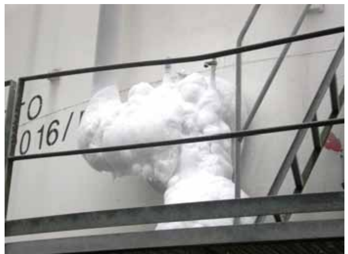
Figure C-9 Valve can no longer be operated
