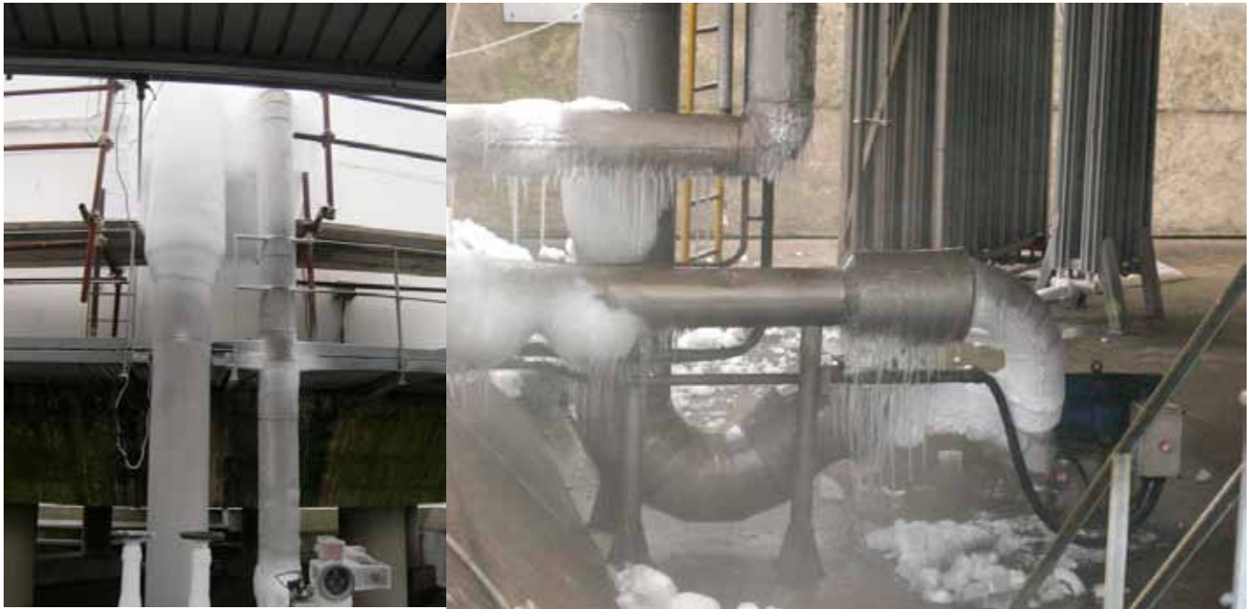
Figure C-11 Broken vapour barriers and insufficient insulation caused ice to form around these pipes causing both process control problems and structural problems
