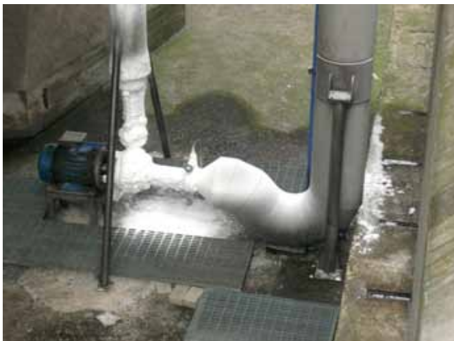
Figure C-8 Pump breaks down
